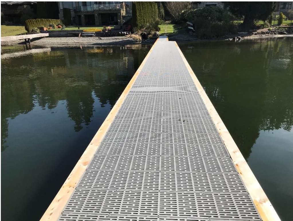
Photo 2. View of pier from end looking east.
